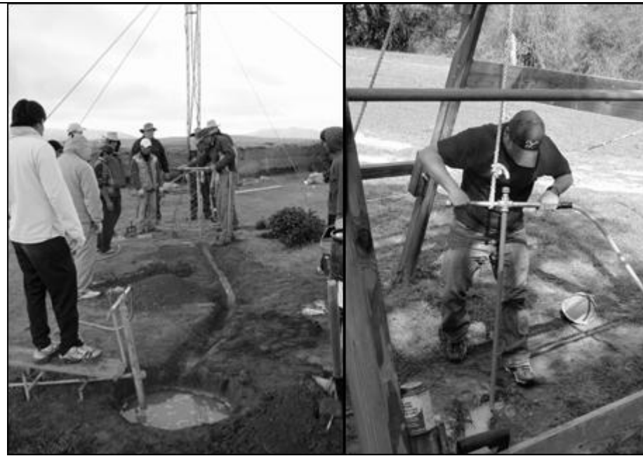
Figure 4: (a) EMAS percussion-jetting set-up, Bolivia [left]; (b) Test-drilling using percussion-jetting at the University of South Florida GeoPark [right] (M. MacCarthy)
