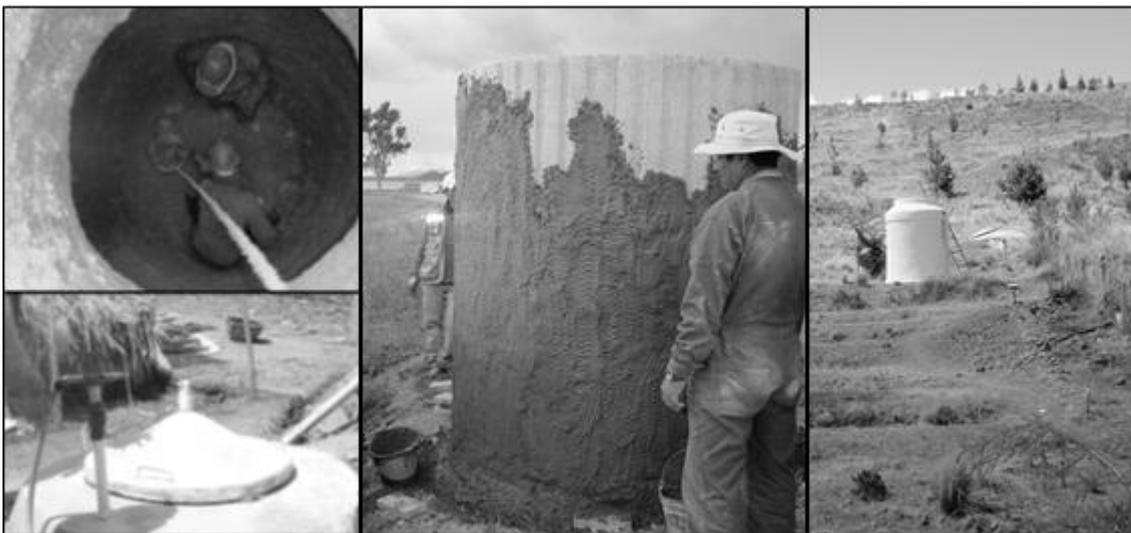
Figure 5: EMAS water storage tanks used in RWHS, (a) underground tank, in construction [top left]; (b) completed underground tank with manual pump [bottom left]; (c) aboveground ferrocement tank, in construction [middle]; (d) ferrocement tank elevated on a hillside [right] (M. MacCarthy)
